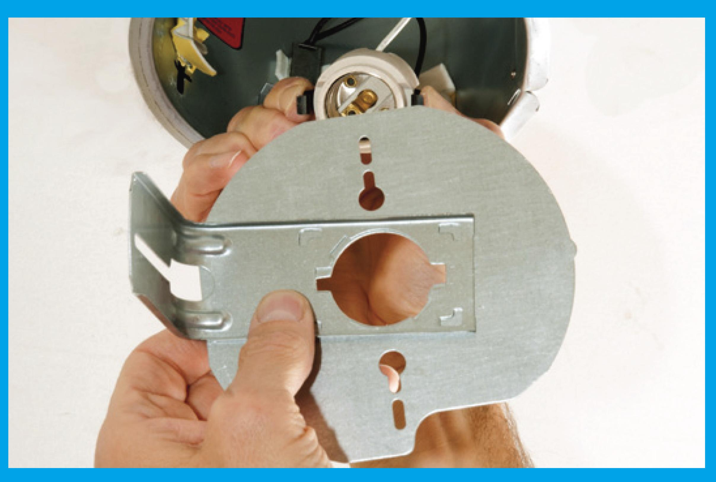
1. Remove and discard the mounting bracket/plate from inside the housing. Place the "Modified Fixture" sticker on the inside of the housing.
