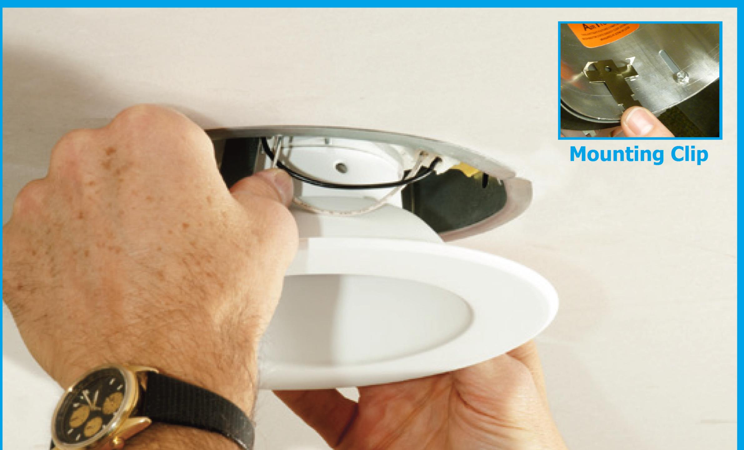
4. Using both hands, squeeze the torsion springs (or v-springs) together while inserting the DLR56 into the housing. Release the springs, allowing them to catch the mounting clips within the housing. Push the DLR56 into the housing and flush with the ceiling.
