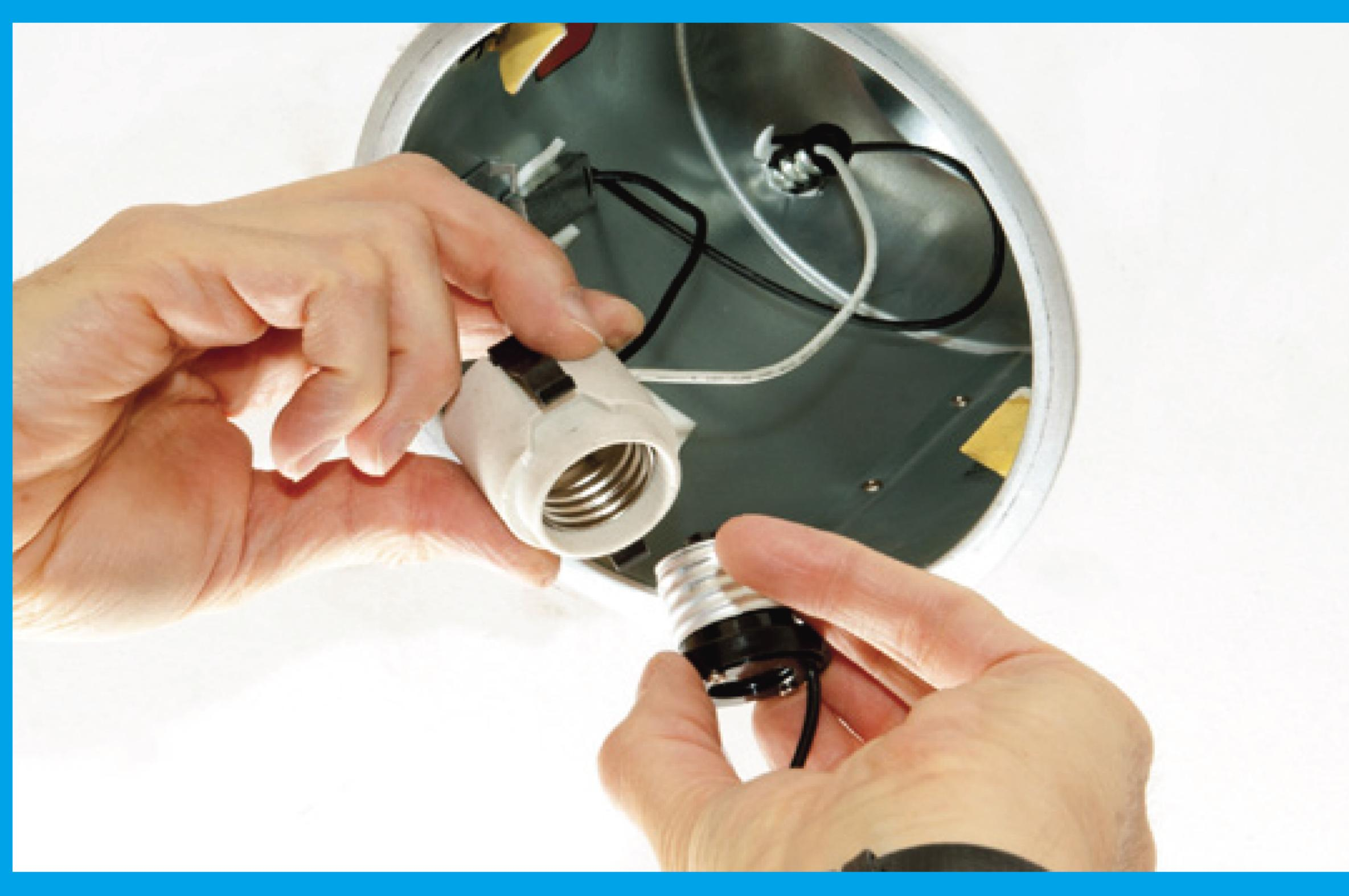
2. Screw in the Edison connector to the Edison base inside the housing. A GU-24 adapter is also available for housings with a GU-24 base.
